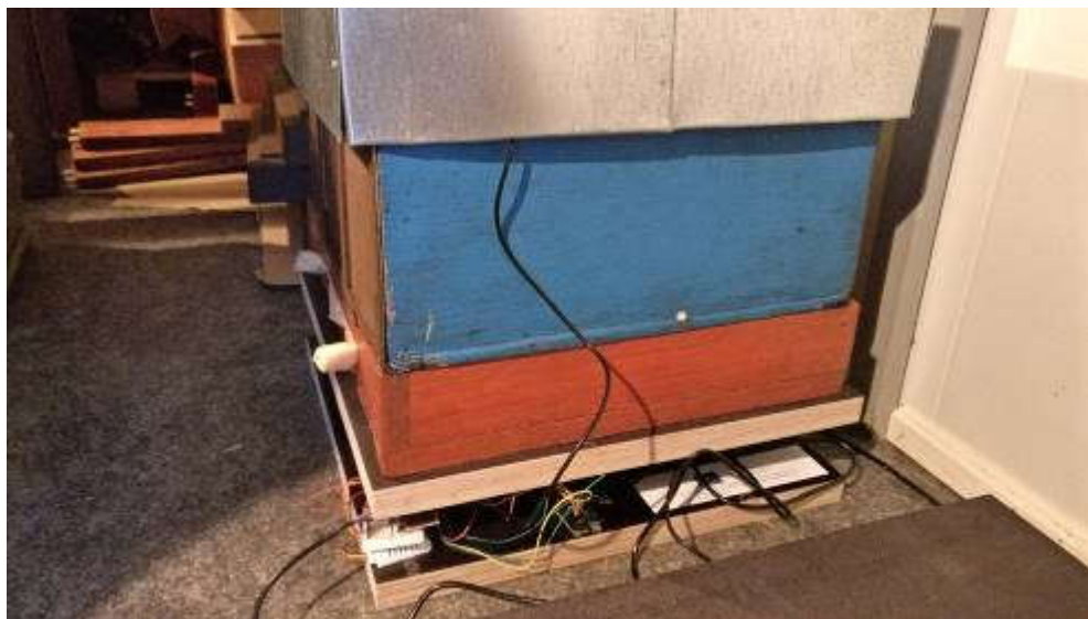
Figure 4. Installation of the system in real environment
