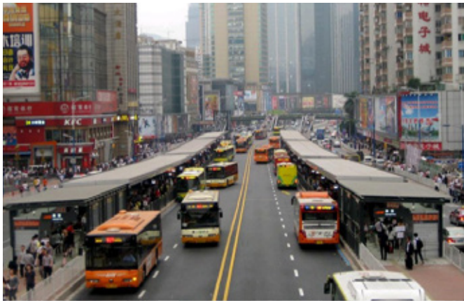
Figure 6. Appearance of the infrastructure after BRT implementation
