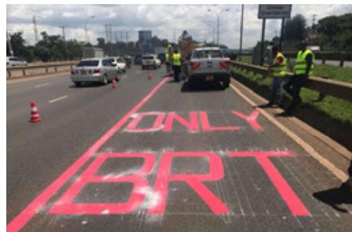
Figure 7. Traffic lane intended for BRT vehicles only
