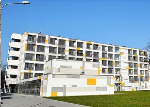
Figure 4. Pavilion 4 - appearance of the constructed building
