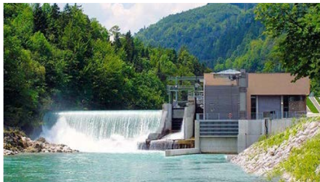
Figure 1. Appearance of a flow-through mini hydro electric power plant, [3]
