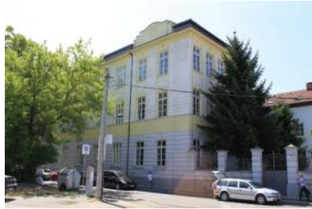
Figure 17. Convent of Sisters of Mercy of Saint Vincent De Paul, Gymnasium. View of main façade and courtyard side from the northwest; present condition.
