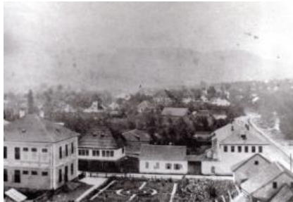
Figure 1. Tsar's school; original site condition. Photograph taken probably after the construction from Ferhadija Mosque's minaret. On the right, western side on the site, beginning of the new section of Kaiserstraße is visible [3]
