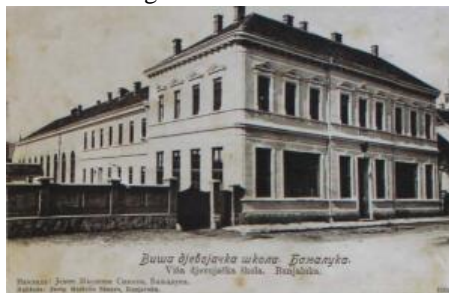
Figure 13. Higher school for girls. View of the northeastern corner. In first plan: main façade with entrance zone. Photograph taken in 1905 [20:74]
