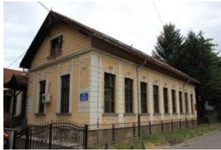
Figure 20. Serbian primary school. View of the southwestern corner; present condition.
