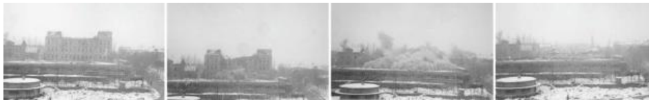
Figure 12. Ober-Realgymnasium; demolition sequence. Photograph taken 1970 [4:193]
