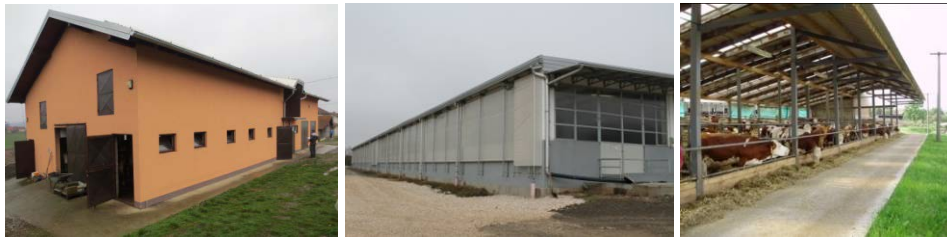
Figure 6. Construction of the peripheral walls of objects for farming dairy cows: closed object, Prnjavor, BH, 2014; semi-open object, Trnopolje, BH, 2014 and open object, Prijedor, BH, 2014 (Source: Authors, left and middle; B. Rogić, right)
