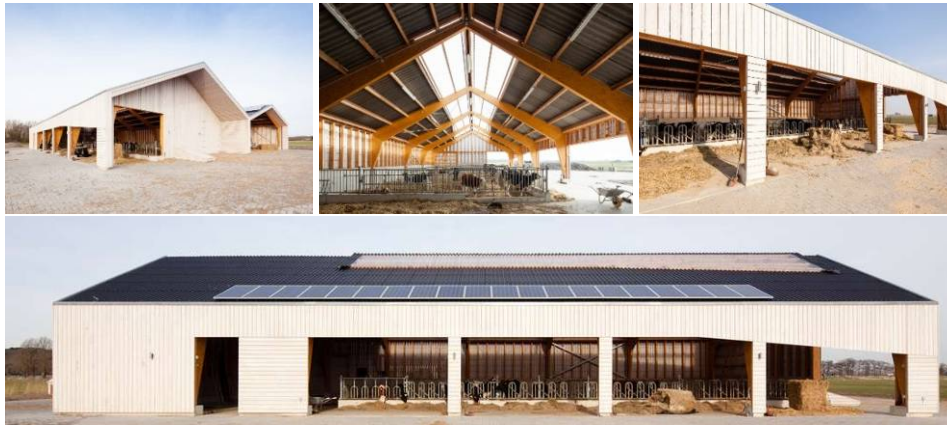
Figure 15. Project „Grote Heklaantje“, Bergen (Netherlands), Negen Graden Architectuur (Source: Architizer)
