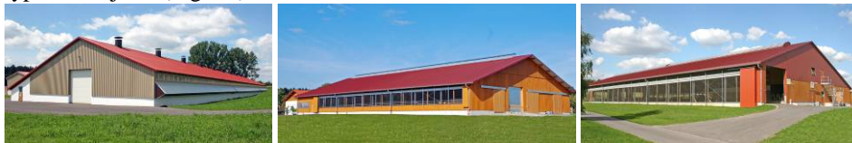
Figure 11. Construction and materialization of the facade walls of modern stables for dairy cows (Source: WolfSystem)
