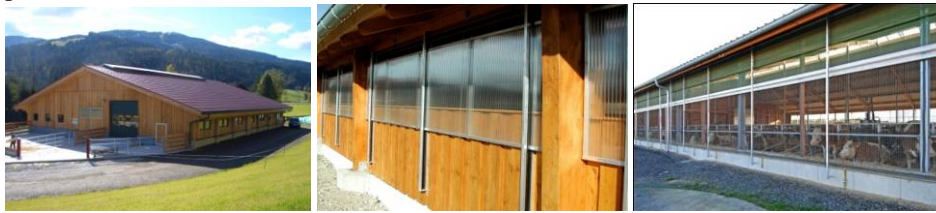
Figure 13. Ventilation and facade lighting in stalls in the EU: in the form of windows, continuous opening above high parapet and completely open facades (Source: WolfSystem)
