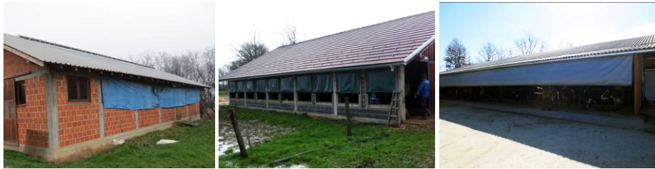
Figure 8. Tarpaulins installed during winter to the open parts of the facade in Bijeljina, BH, 2014 (left); Gradiška, BH, 2014 (middle); and Prijedor, BH, 2014 (right) (Source: Authors)
