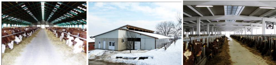
Figure 9. Zenital lighting through: transparent roof elements, Czech Republic, 2009; openings created by the skimming the roof level, Kozarska Dubica, BH, 2014 and lantern, Trnopolje, BH, 2014, left (Source: Authors)
