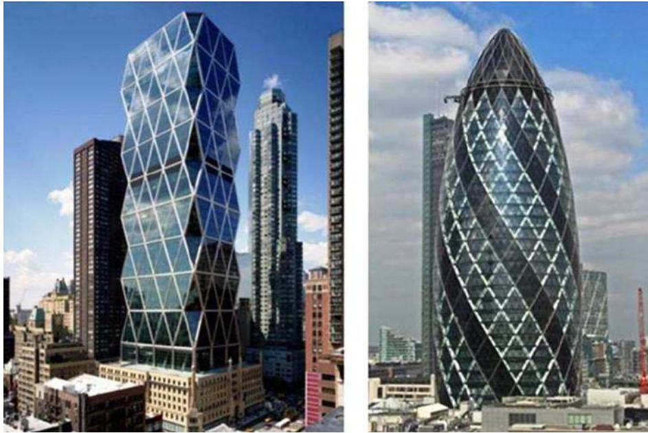
Figure 11. Hearst Headquarters Centre in New York (left), and 30 St. Mary Ave in London (right) [12,13]
