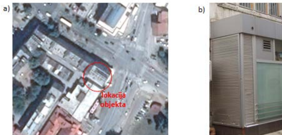
Figure 4. a) location of building, b) chamber enclosing the exterior units of the air-conditioning system
