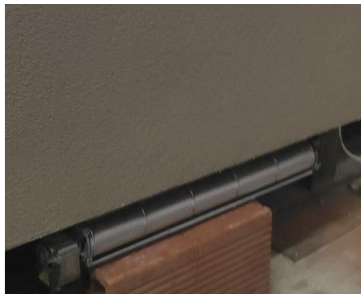
Figure 3. Cross flow fan under the PCM section.
