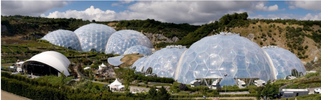
Figure 8. The Eden Project, Cornwall, UK (arch. Nicolas Grimshaw, 2001), the largest public/botanical greenhouse in the world. The envelope is comprised of hexagonal-triangular tubular steel structure, covered with inflated panels made of ETFE (ethyltetrafluoroethylene). [21]
