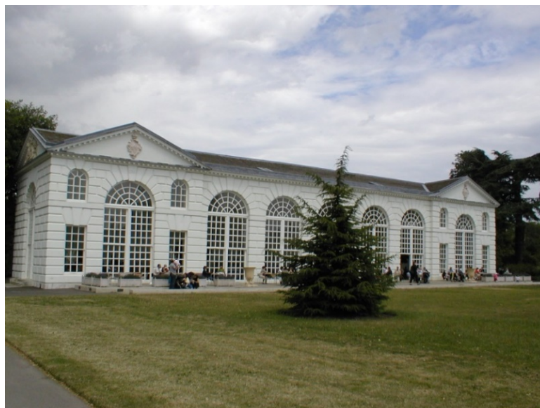
Figure 7. Orangery at Royal Botanical Gardens Kew (arch. William Chambers, 1761), now serves as a restaurant. [19]
