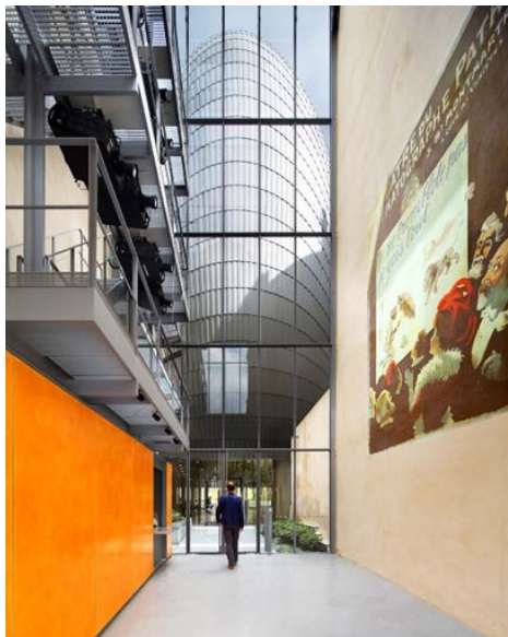
Figure 4. Pathe Foundation, Renzo Piano, Paris, France: Main public entrance to the Foundation (1)
