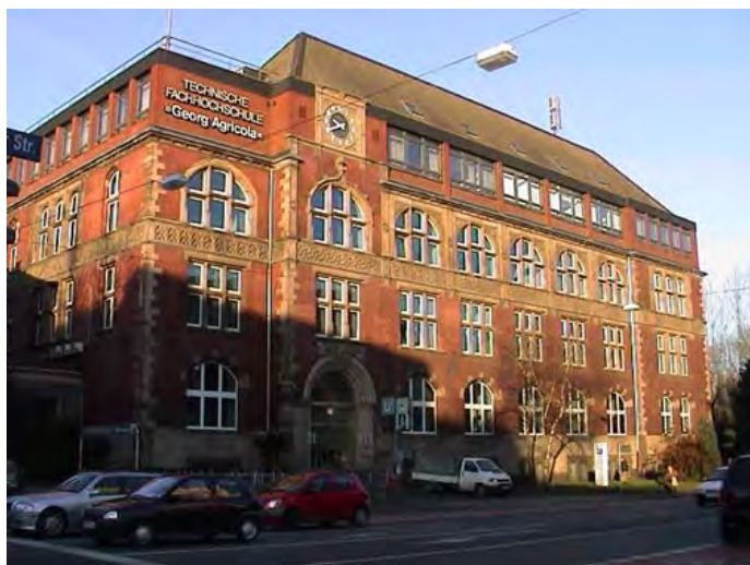
Fig. 1: the Georg Agricola University of Applied Sciences main building
