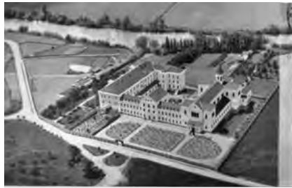
Figure 3. Mariastern Abbey; view of the new complex. [18:121]
