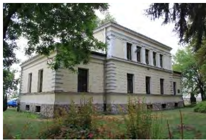
Figure 13. Evangelistic Parish house. View of the main façade from the northwestern corner; present condition. [18:151]
