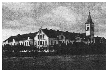
Figure 7. Convent Nazareth with belonging facilities; photograph dated in years before WWII [18:133]
