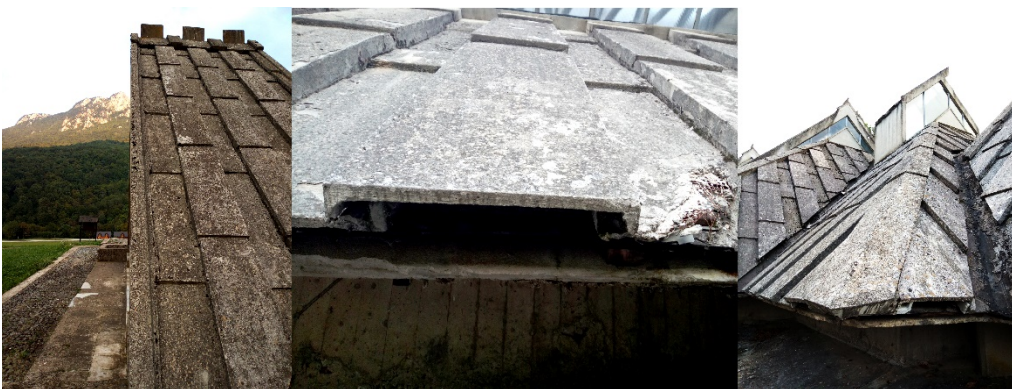
Figure 5. Brutalist interpretation of roofing patterns—landscape references (left), a detail of tile overlay (in the middle), roof hip details (right) (source: Marina Radulj)
