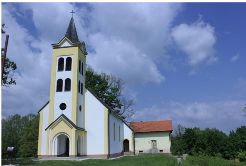
Church of Saint Michael the Archangel, Čelinovac: view from the south
