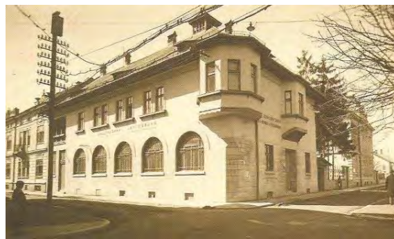
Figure 10. Landesbank branch; view of the northeastern corner [8:193]
