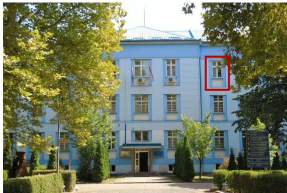
Figure 3. View of the western façade with the main entrance to the Rectorate building. The examined room is the uppermost right in the view, as indicated on the image.
