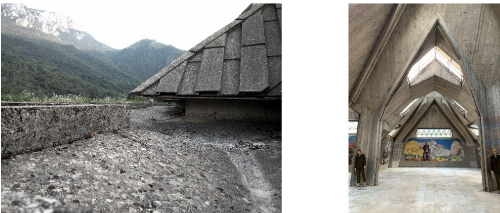
Figure 2. Left: a detail of the overhang and the wide drain around the Memorial House; proportions of a Japanese temple (source: Marina Radulj) Right: basilical and constructivist interior of the Memorial House (Jen Lukehart retrieved from https://www.sosbrutalism.org/cms/19405697 on 27 October 2021)
