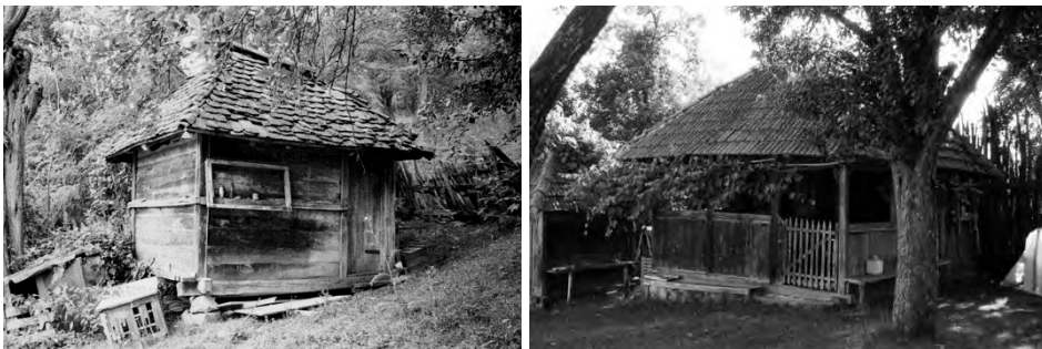
Fig. 14, 15. Vajat with skeleton and filling of planks connected "na unizu" (village Brajkovići) / Magaza with porch (village Mionica).
