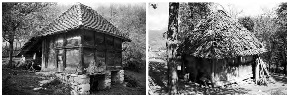
Fig. 5, 6. Magaza covered with clay tiles (village Makovište) / Magaza covered with wooden shingles (village Makovište)
