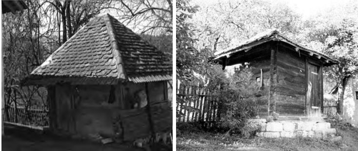
Fig. 12, 13. Vajat in planks "na unizu" (village of Brajkovići) / Vajat in planks "na čert" (village Mionica)
