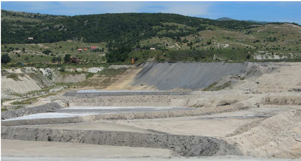
Picture 2. Internal disposal site of electrofilter ash (Cassette I i II)
