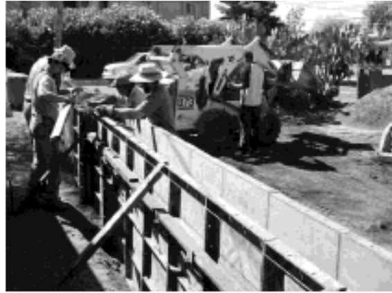
Figure 5. Placing and ramming in wall forms
