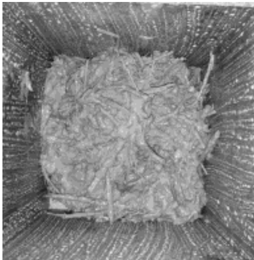
Figure 6. Placing of light clay
