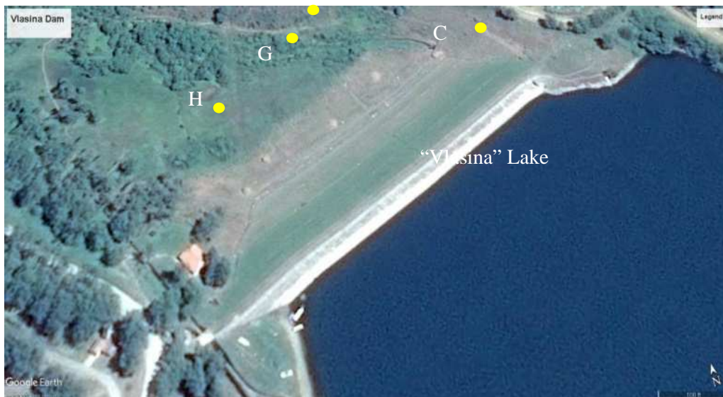
Figure 3 “Vlasina” dam and positions of pillars for dam monitoring
