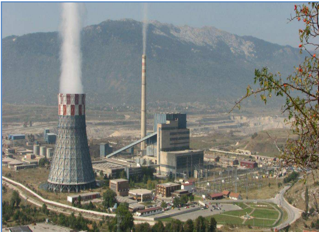
Figure 1. Thermal Power Plant Gacko [8]
