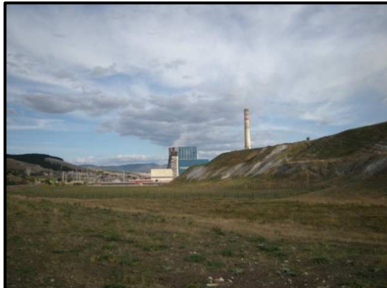
Figure 3. Power plant Gacko and dumps in the process of recultivation [14]
