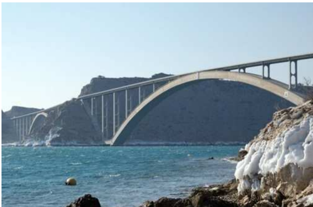
Figure 2 Large concrete arch bridge near the island Krk in Croatia whose lifetime should be several hundred of years
