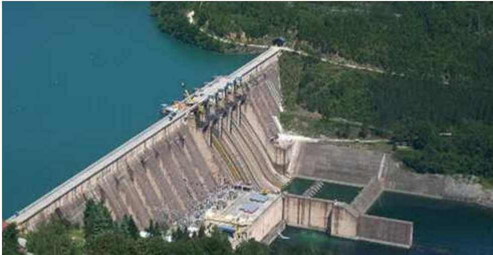
Figure 3 Hydro power plant on the river Drina
