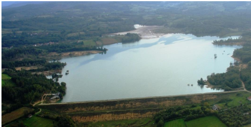
Picture 3. Dam and tailing storage facility
