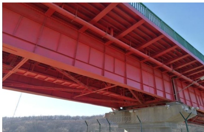
Figure 1 Bridge span over the Vorona River in Borisoglebsk
