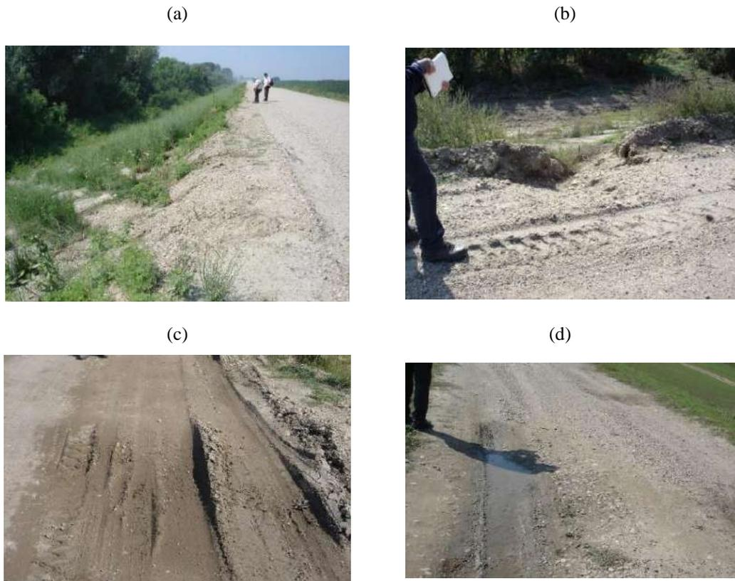
Figure 11 Registered types of deformations on the embankment: (a) Type I of deformations: overflow of the added sand-gravel material over the basic embankment; (b) Type II deformations: gutters - erosion furrows along the perimeter of the embankment crown; (c) Type III deformations: depressions on the road; (d) Type IV deformation: holes in the crown of the old embankment.
