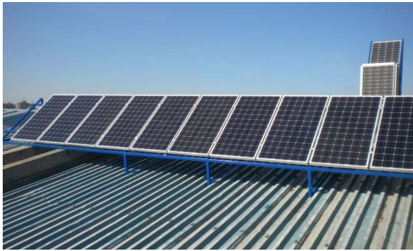
Figure 1. Solar power plant power of 2 kW on the roof of FSM in Niš
