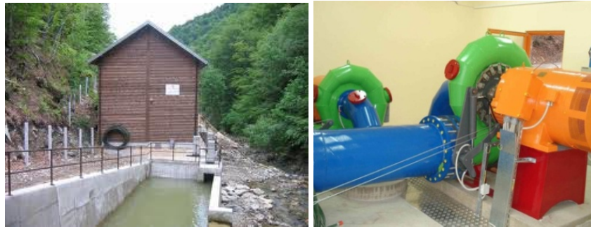
Figure 6. An example of a small hydroenergy plant [20]
