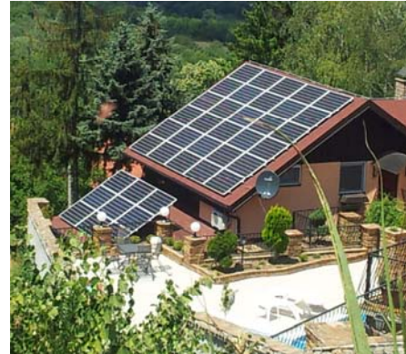
Figure 12. PV solar plant of 10 kWp in the village of Cortanovci
