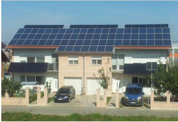
Figure 11. PV solar plant of 20 kWp in Belgrade
