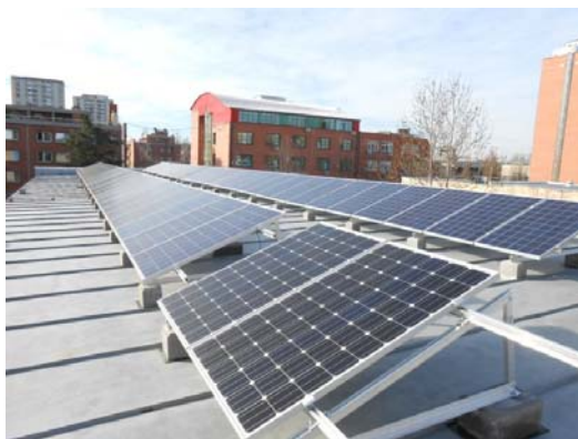
Figure 5. PV solar power plant FTS2 of 15.9 kWp on the building of the Faculty of Technical Sciences in Novi Sad
