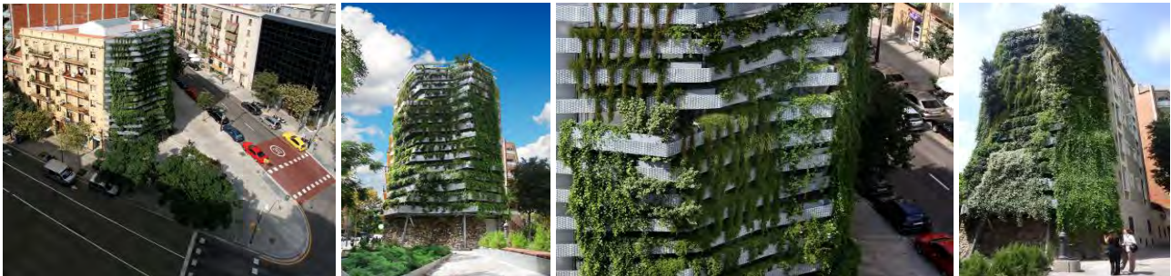
Figure 1. „Vegetecture.” The 69-foot wall is green grows where Galvanized steel scaffolding Garden Tarradellas. Mediatrix Green vertical garden. Capella Garcia Arquitectura Rather queasily call this project in Barcelona, [16–18].
