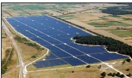
Figure 7. The biggest photovoltaic power plant in Bulgaria – Karadzhalovo . [20]
