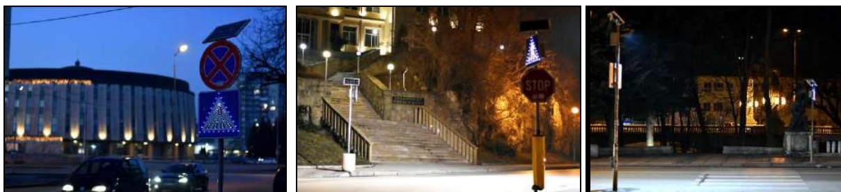
Figure 17. PV-LED systems for additional illumination of road signs and pedestrian walkways
