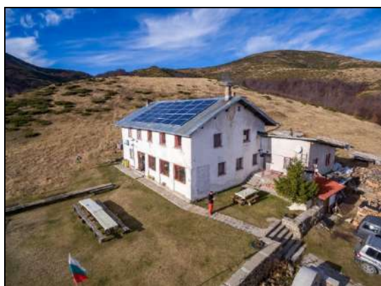
Figure 18. Autonomous PV system for power supply of high-altitude mountain information center Tazha hut in National Park „Central Balkan“ [30]
