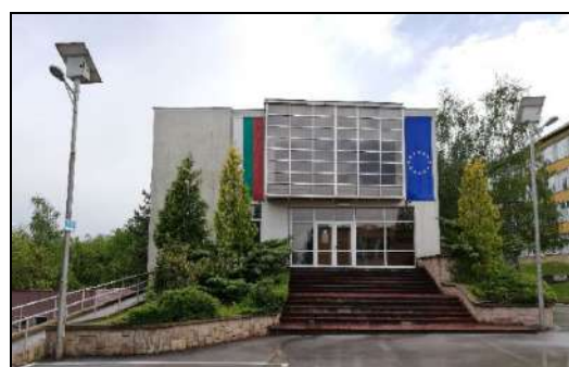
Figure 16. PV-LED system for external lighting at the Technical University of Gabrovo
