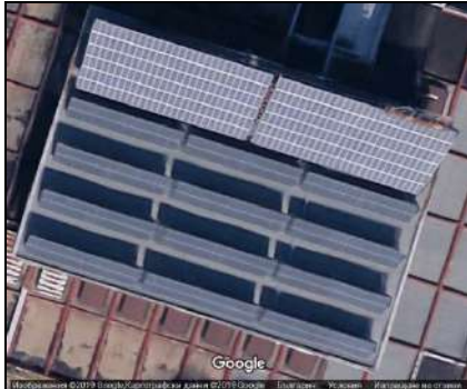
Figure 10. Satellite photo (Google) of 132 kWp roof-mounted solar power plant in the industrial enterprise ZITA. [23]
