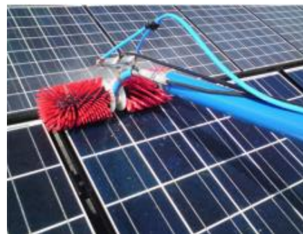
Figure 6. Cleaning solar modules with water under pressure and brush [26]
