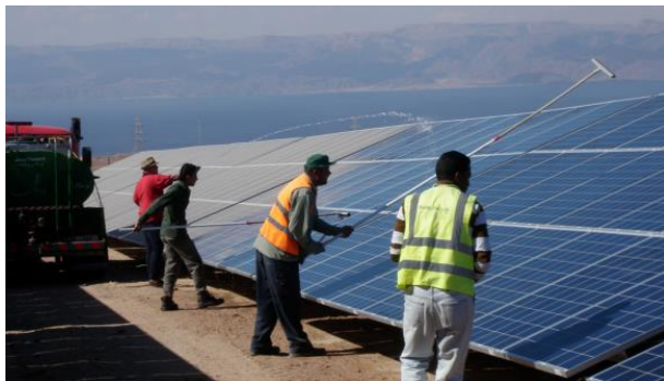
Figure 5. Manual cleaning of solar modules [25]
