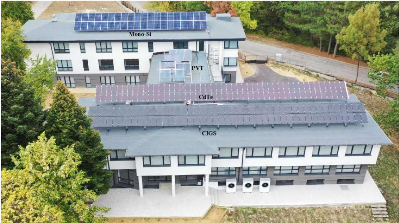
Figure 2. Disposition of the three PV power plants on the roof of the Competence Center building at the Technology Park of the Technical University of Gabrovo, Bulgaria
