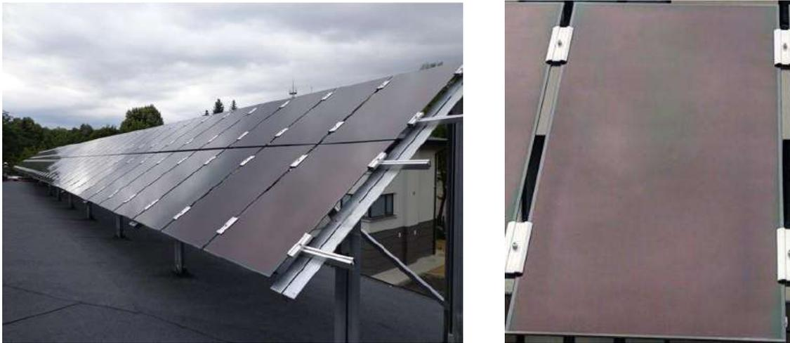
Figure 5. CdTe PV modules power plant
