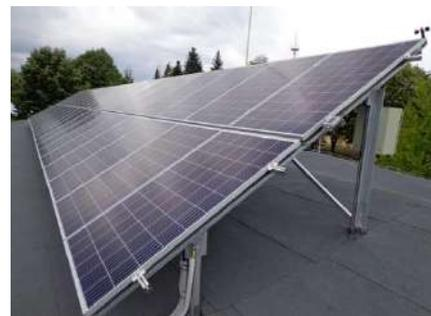
Figure 3. Mono-Si PV modules power plant
