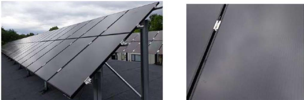
Figure 8. CIGS PV modules power plant
