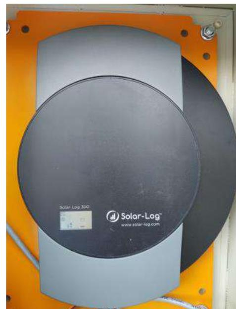
Figure 11. The monitoring system of the PV power plants with model Solar-Log 300
