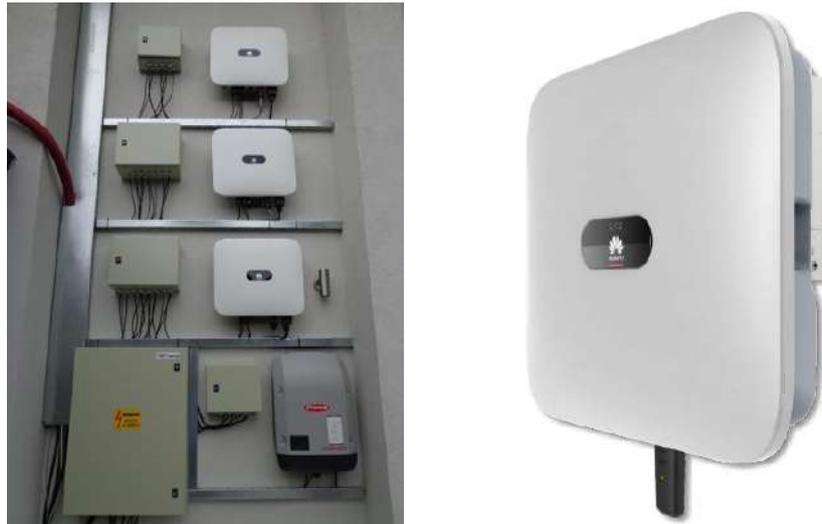
Figure 10. Disposition of the three-phase grid-tied PV string inverters and appearance of the model SUN2000-10KTL-M0
