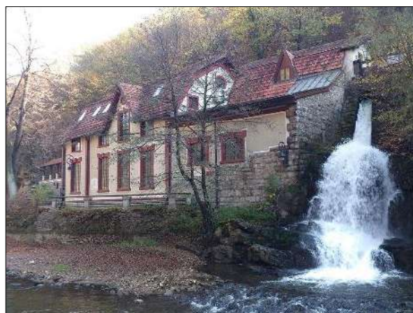
Figure 1. SHP Pod Gradom, Užice, 1900.
