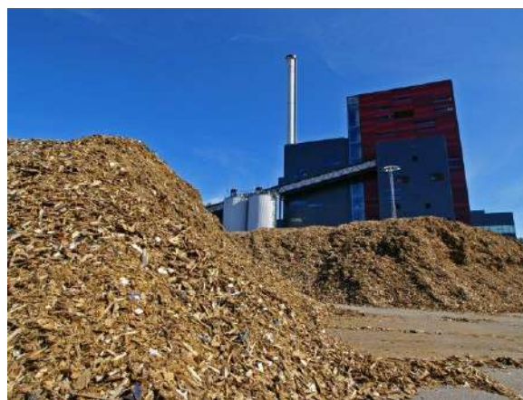
Figure 21. Pellet and biomass power production plant, Boljevac, 2021. [8]
