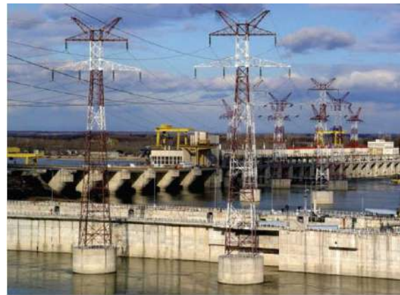
Figure 4. Hydropower plant Đerdap II, Kusjak, Negotin, 1985.
