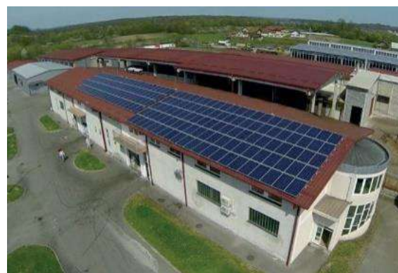
Figure 18. PV solar power plant MI Trivas Ltd. of 50 kWp, Prnjavor, 2014/15.
