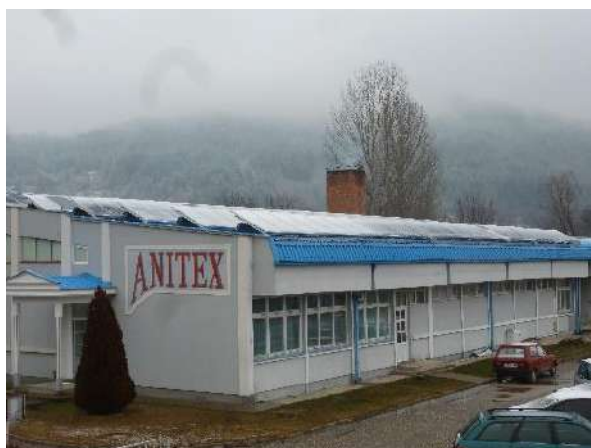
Figure 15. PV solar power plant Anitex, 40.32 kW, 2013, Bosilegrad (Plan-net-solar, Slovenia)
