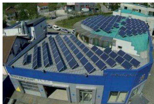
Figure 19. 48 kWp PV solar power plant of the company Verano Motors from Banja Luka, 2013.
