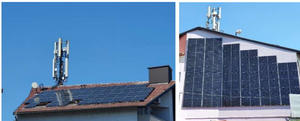
Figure 12. Photovoltaic modules on the roof and the facade of the building
