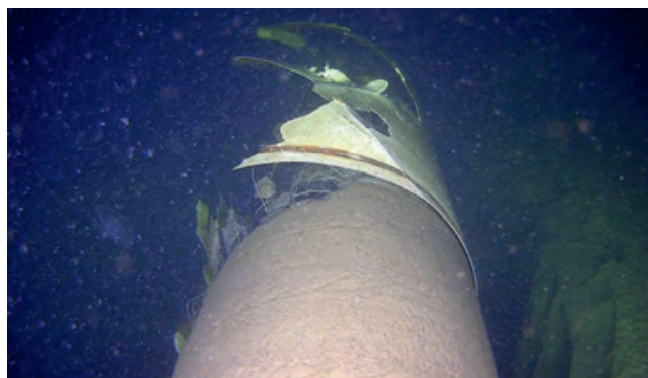
Fig. 3. The damaged offshore Balticconnector gas pipeline. Source: [8]
