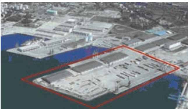
Figure 1. The container and general cargo terminal at the Port of Bar (Source: web)
